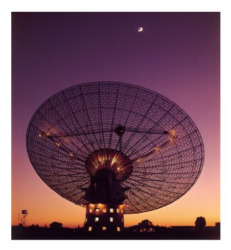
Also mentioned was 64 metre Parkes Radio Telescope in Australia that received signal from the Apollo 11 lunar landing whilst experiencing high winds (peaking at 62mph) above its design limits.
